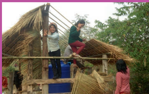
A roof being constructed over the bio-sand water filtration system
