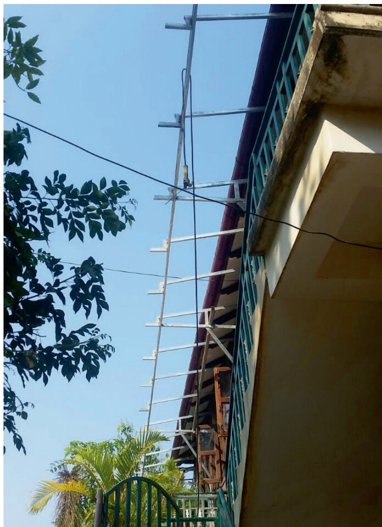
Constructing the roofing and gutters to prevent leakage
