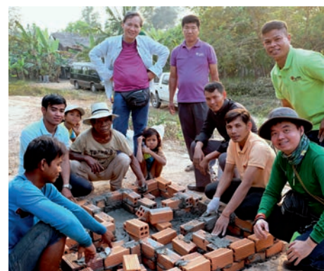
Caritas Siem Reap and local villagers building the base for the Bio-sand Water Filtration System
