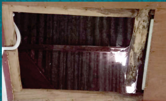
Deteriorating roof with holes of St. Elisabeth Boarding House in Bondo Kodi - Sumba Indonesia.
