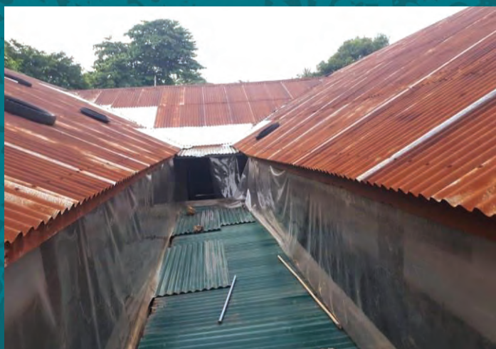
Deteriorating roof with holes of St. Elisabeth Boarding House in Bondo Kodi - Sumba Indonesia.
